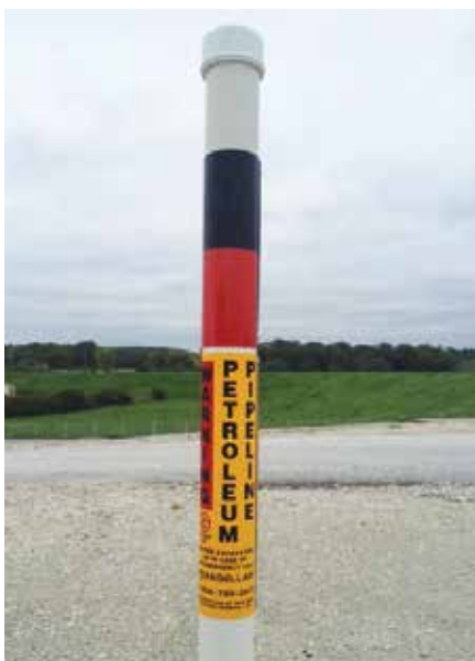
Our pipeline markers can be typically identified by the black and red bands at the top.
